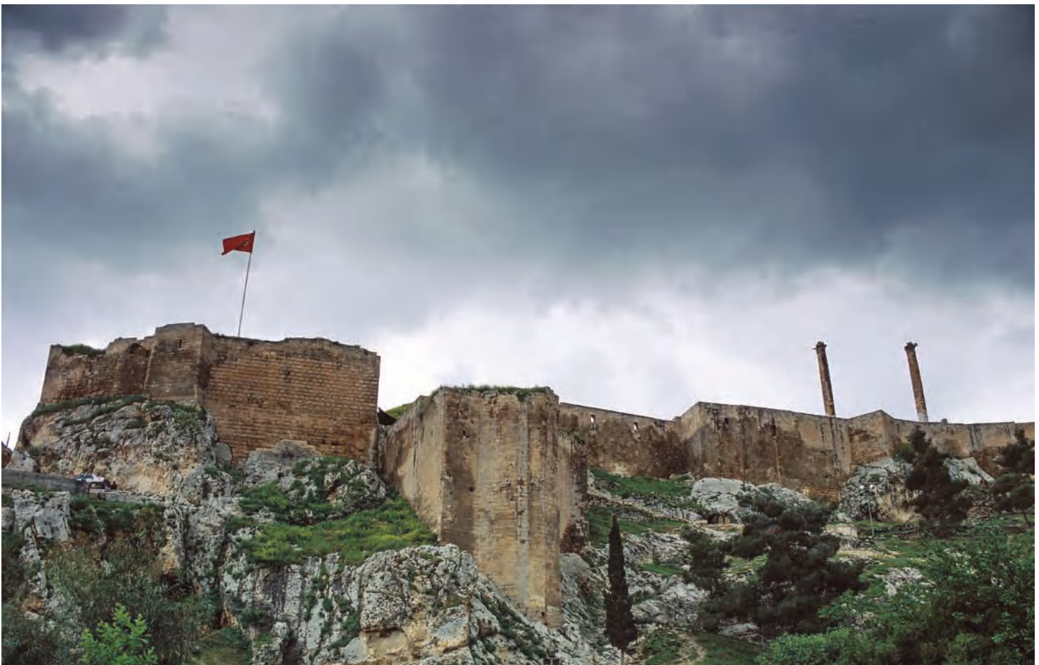
96. The city of Edessa, today Şanlıurfa in south-east Anatolia, was conquered by Tigranes II around 83–80 BCE. In the picture, the crusader castle and on the right two columns of a Roman temple. Photo 2001.
