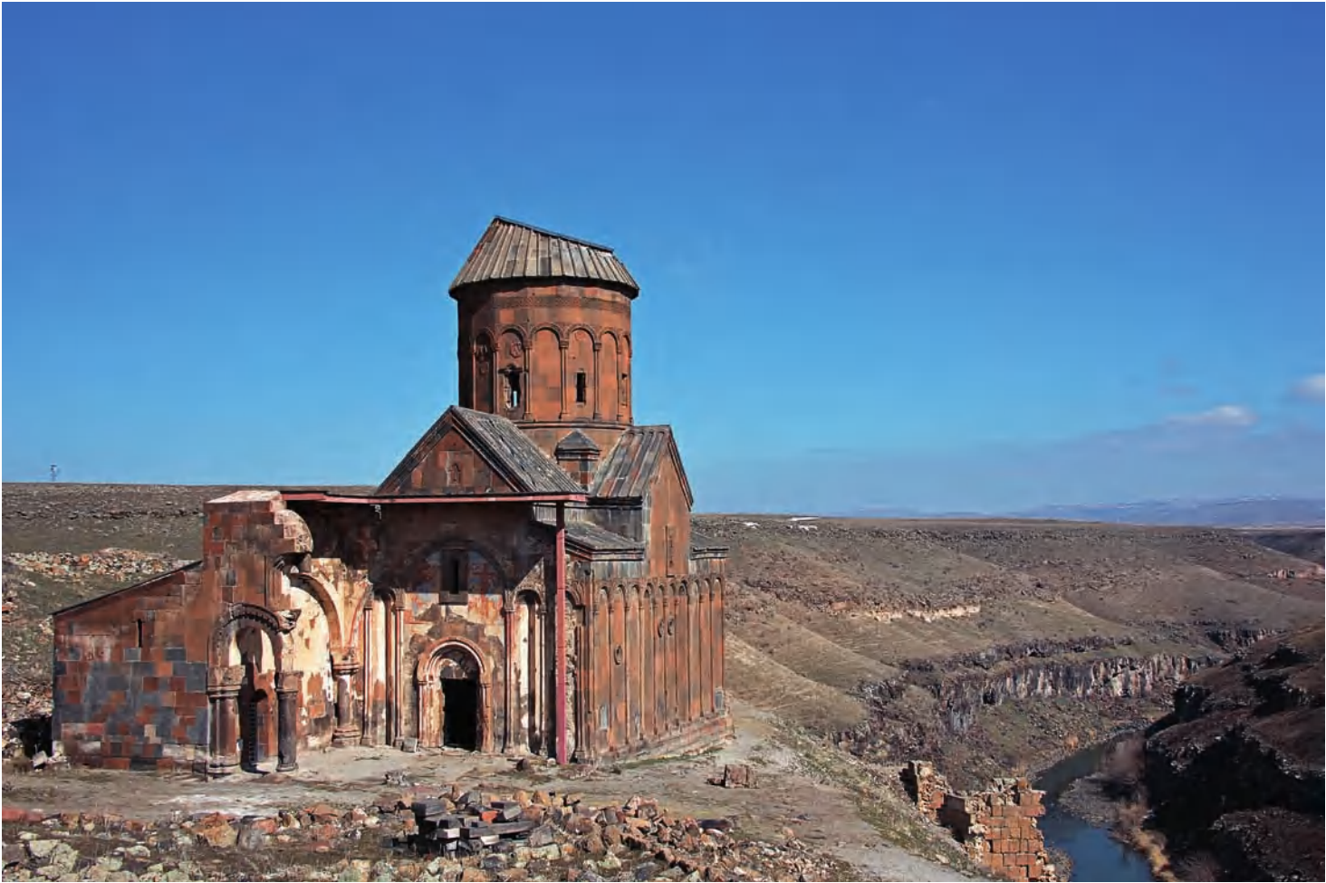
208. The church of St Gregory, founded around 1215 by the merchant Tigran Honents in Ani; on the right in the picture is the River Achuryan, which here forms the border between Armenia and Turkey. The gavit in front of the church has collapsed. Photo 2016.
