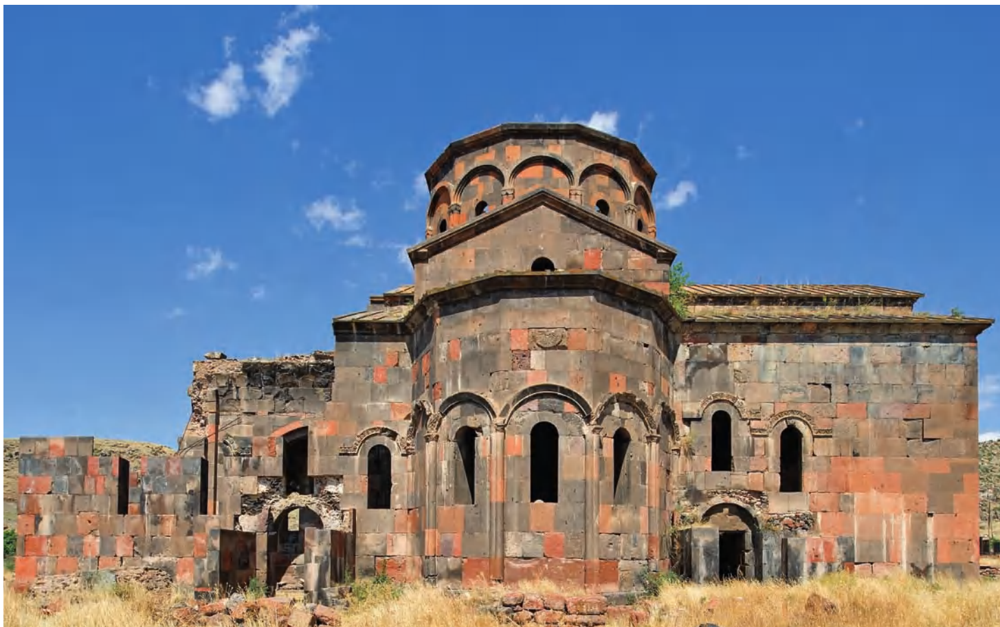
170. The cathedral of Talin from the seventh/eighth century, Armenia, founded by the Kamsarakan dynasty. The cathedral is a combination of a three-nave basilica, a central building and three semicircular conches. In the apse, there are traces of murals from the period of construction. Stone material from the cathedral was used to build the small neighbouring Church of Our Lady. Photo 2015.
