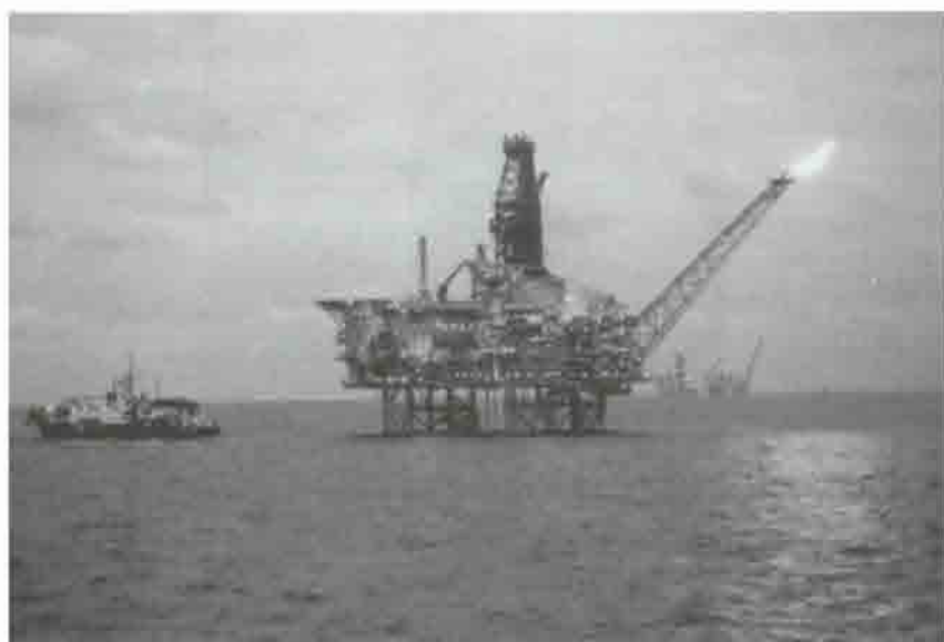
The West Azeri platform, developed and operated by BP/AIOC in the Azerbaijani sector of the Caspian Sea
