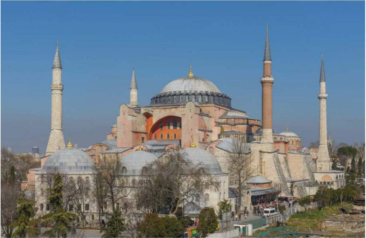
Figure 4.3 Aya Sofya, Exterior.
