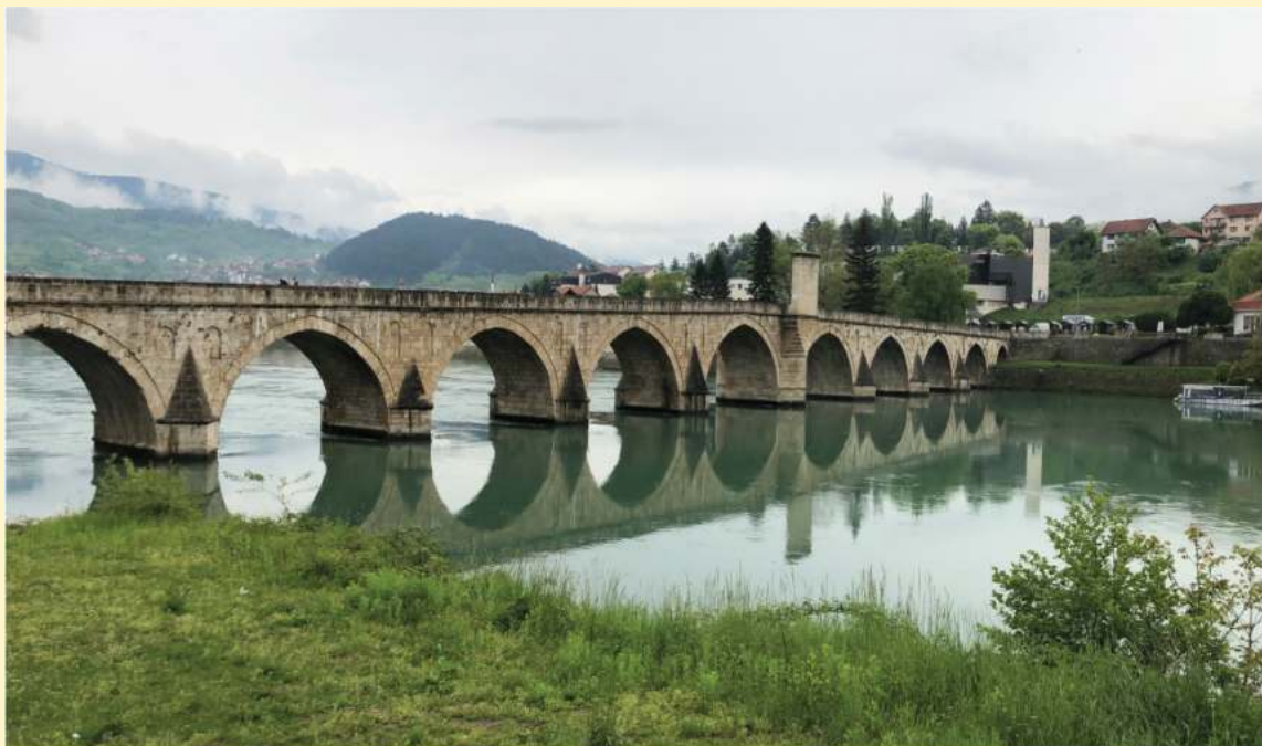
Figure 8.3 Mehmed Sokullu Bridge over the Drina River, Bosnia.
