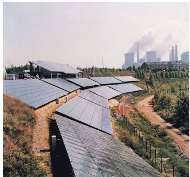
Fig. 2.47 Solar cell field as competition to coal power stations in the background
