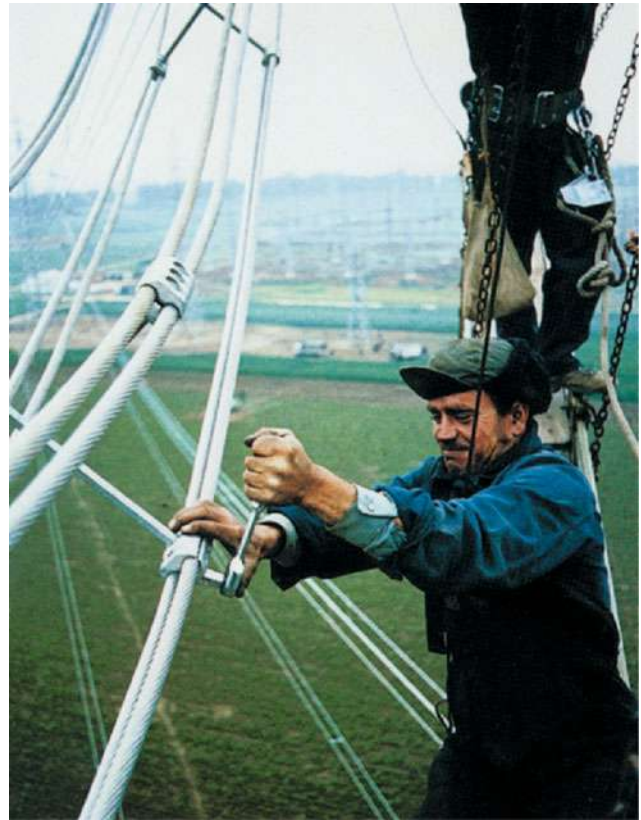
Fig. 5.37 Installation of a high voltage power line. In this picture each phase of the three phase current is transmitted by 4 cables arranged in quadratic form, connected by the diagonal bracket seen in the upper part of the picture. Each cable consists of two wires. The technician just fixes the connection between these wires (with kind permission by information center of the Elektrizitätswirtschaft Frankfurt)
