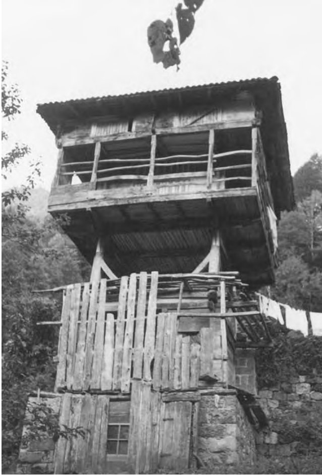
Figure 8.4 A traditional food store serender (also called nalya in Hemshin) in the Makrevis mahalle. Two important characteristics of these stores are their very good ventilation and fixed discs on each wooden column – here galvanized iron plates are used for the same function – to protect the stored foods from rodents.
