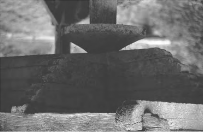
Figure 9.9 Lisers on the tops of poles designed to keep mice out of the serender.
