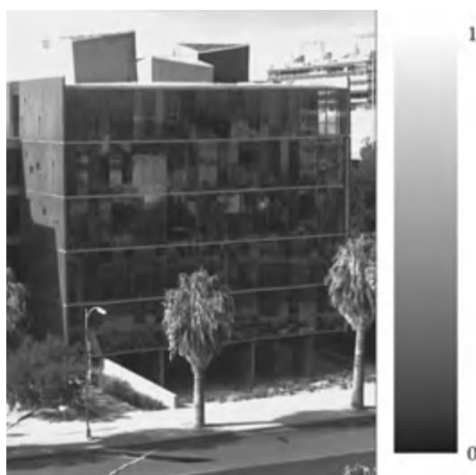
Figure 3.7 An intensity image of the University of Arizona's Meinel Optical Sciences building. The entire north face of the building is windows tilted at various angles. The top of the football stadium is seen at the upper right. High intensity is white, and low intensity is black.
