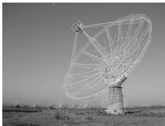
Fig. 3.8 Fully steerable 45 m paraboloidal dishes of the Giant Metrewave Radio Telescope (GMRT) in Pune, India. The GMRT consists of 30 dishes of 45 m diameter with 14 antennas in the central array. Photograph courtesy: Professor Govind Swarup, GMRT, Pune. A color photograph appears in the insert at the back of the book.
