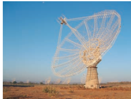
Chapter 3—Fig. 3.8 Fully steerable 45 m paraboloidal dishes of the Giant Metrewave Radio Telescope (GMRT) in Pune, India. The GMRT consists of 30 dishes of 45 m diameter with 14 antennas in the central array. Photograph courtesy: Professor Govind Swarup, GMRT, Pune.
